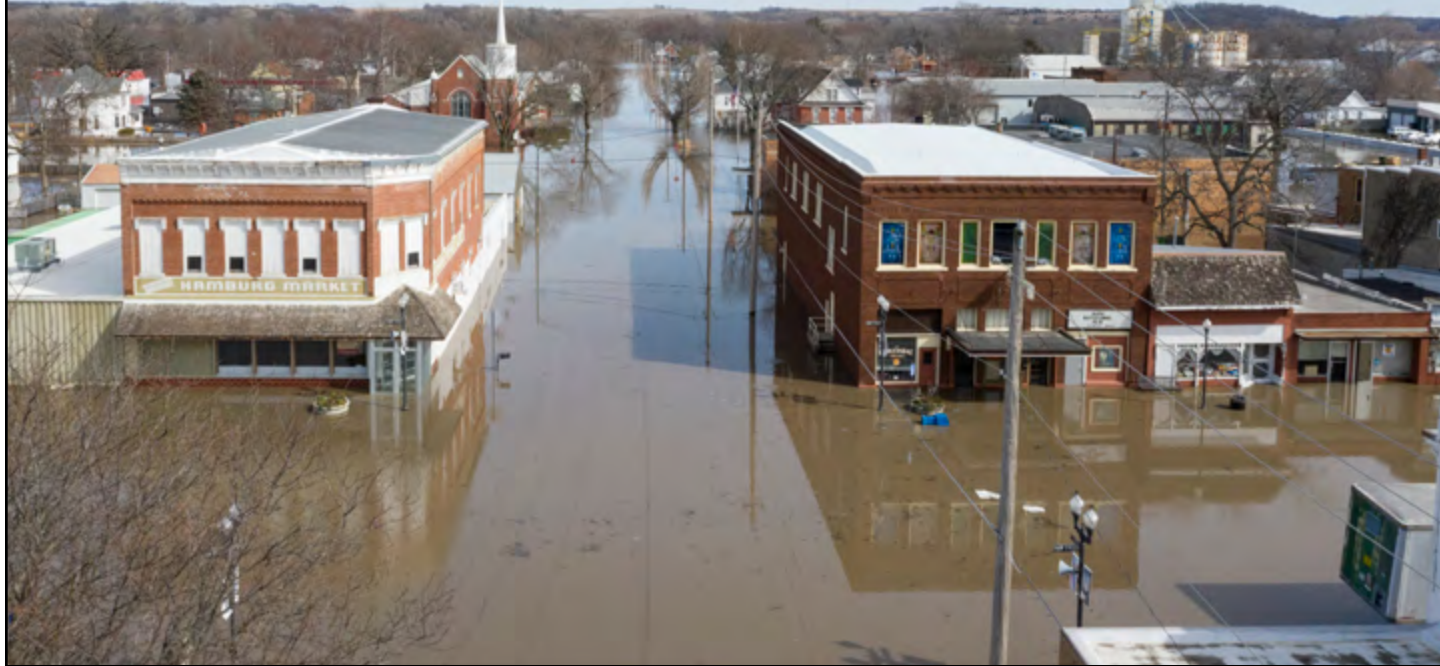
Floodwaters of the Missouri River spread across the town of Hamburg, Iowa, in March 2019. The town experienced three flood events between March and September this year. Residents rebuilt the levee in May, which helped when the river crested at 22 feet in September. (Photo courtesy of Jenn Ackerman and Tim Gruber for The New York Times)
