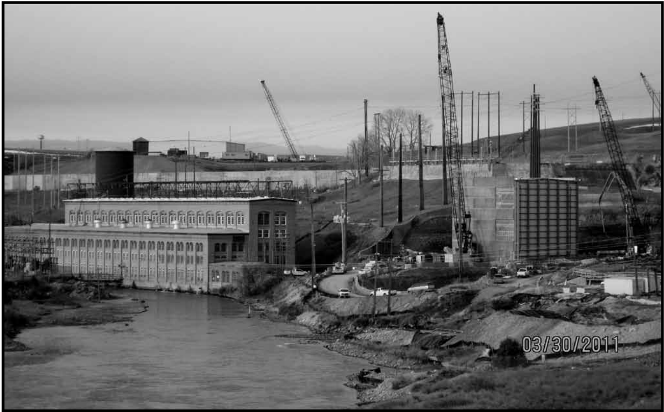
Old powerhouse and construction of new powerhouse. Photo: Chris Dantic
