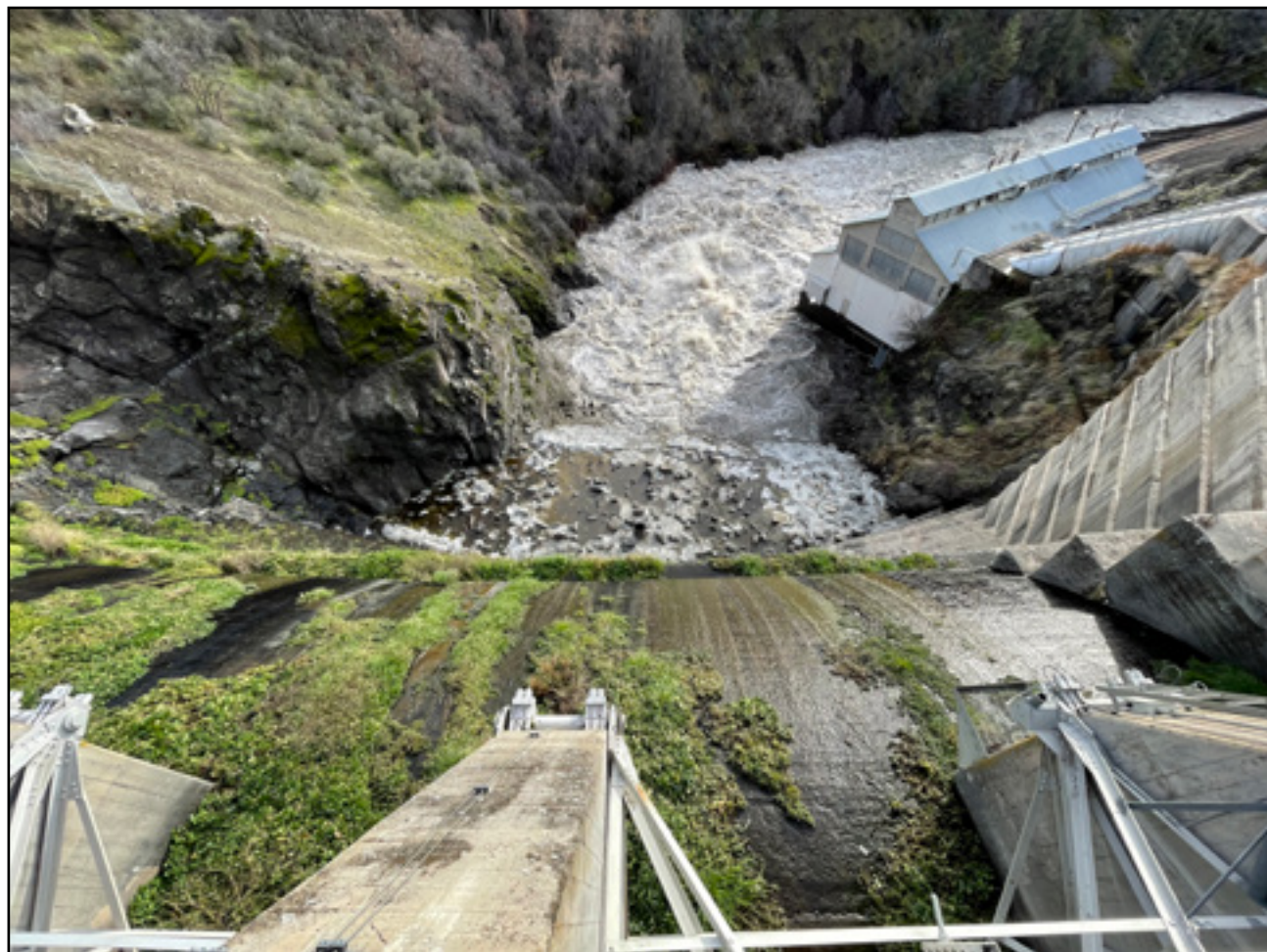
Copco Dam was the last to be breached when a blast at the base of the structure unleashed 4,000+ cfs.
