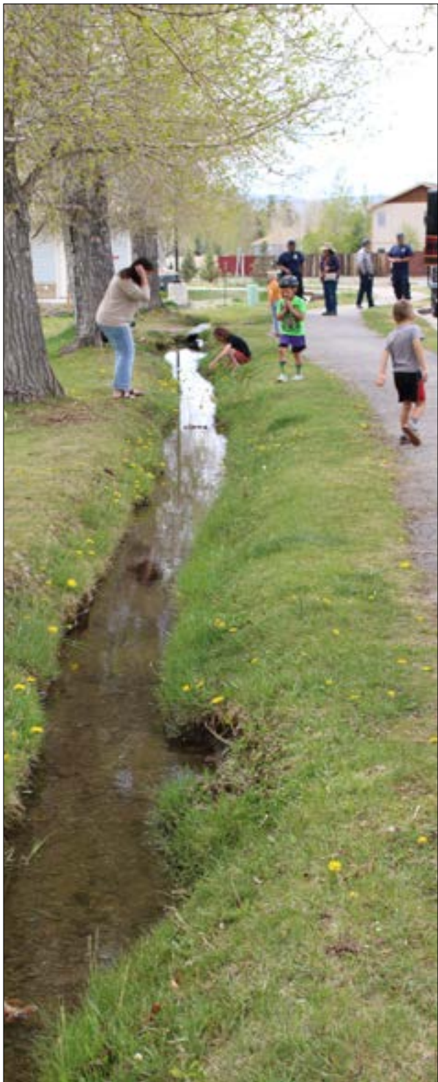
Debris-Free Drainage: A well-maintained irrigation ditch carries irrigation water through the town of Gunnison.
