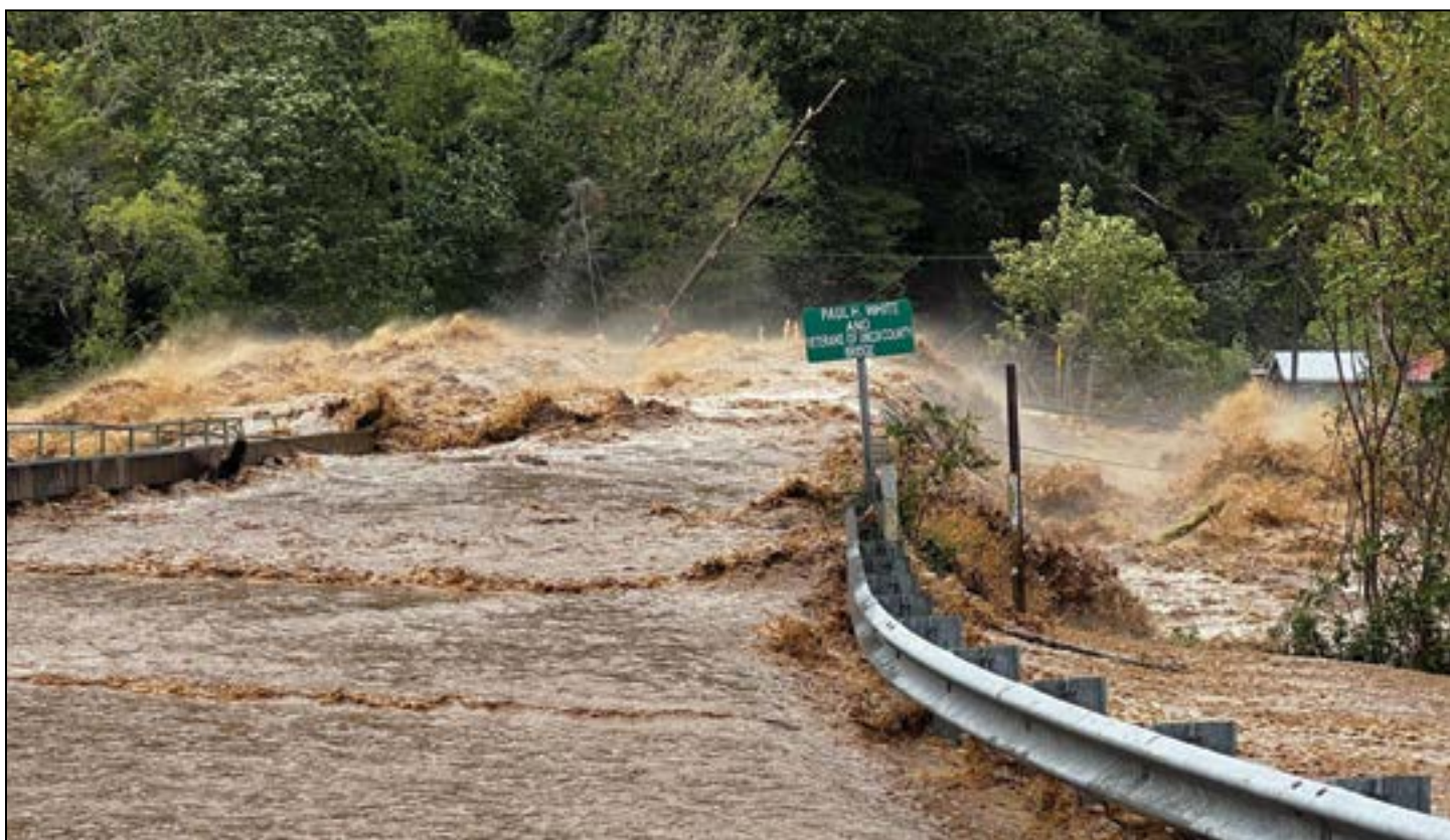
Bridge Before Collapse: Bridge on Nolichucky River in Unicoi County, Tennessee, washed away during Hurricane Helene in 2024. Photo: Trey Moore
