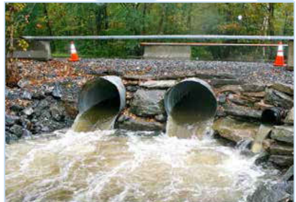
The Town of Becket used the opinion of probable costs and conceptual designs, funded by the Committee, to leverage an additional $399,000 in grant funds to replace this road-stream crossing with a fish-friendly, flood resilient structure. The road-stream crossing had washed out two times in less than six years.
