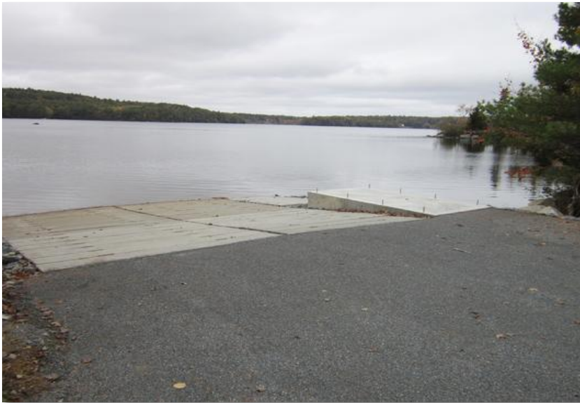
Walker Pond boat launch with concrete abutment at right
