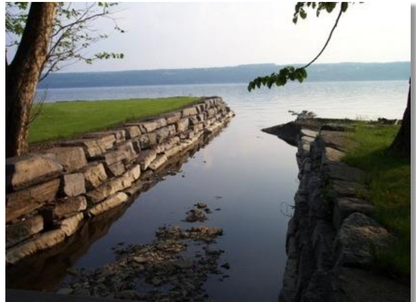
Stone bulkhead launch wall
