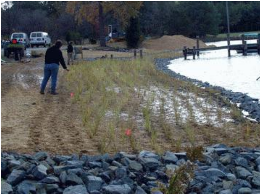
Natural buffering system called low stone sill helps to reduce wave impact while newly planted native grasses re-establish a fringe marsh.
