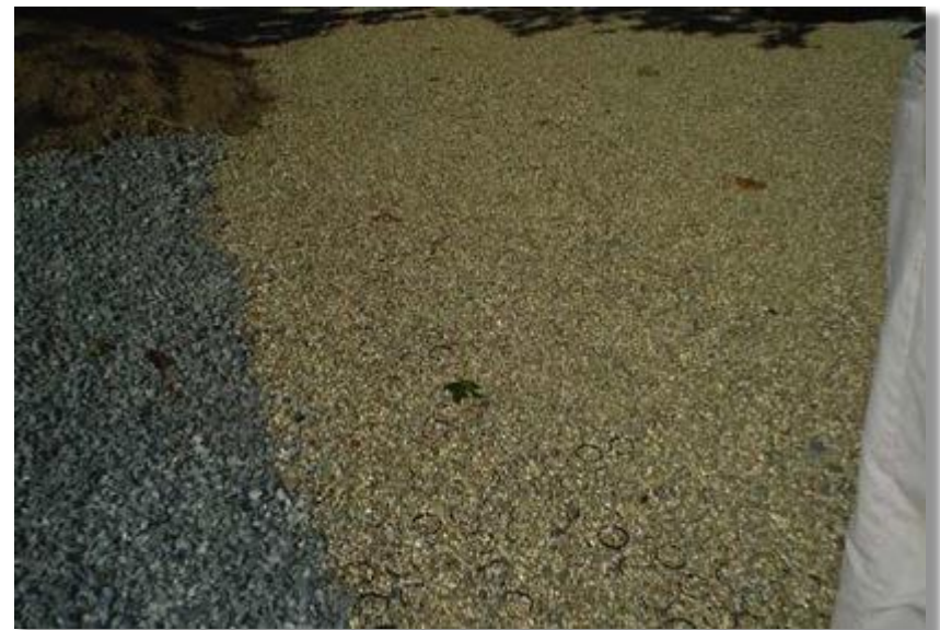
Gravel (on right) adjoins aggregate
