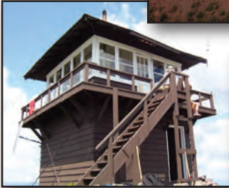
COVERED WITH STRUCTURE PROTECTION WRAP
