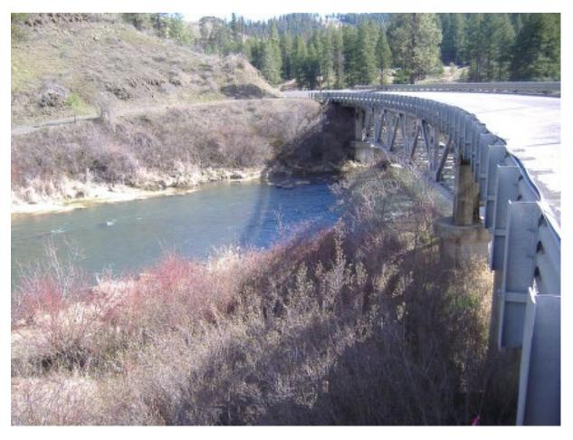
Existing Bridge was a 285-foot (ft) long bridge. The approach spans consist of reinforced concrete deck girders and the center span is a 150-ft long truss and includes 1 bent within OHW and 1 partially within the OHW
